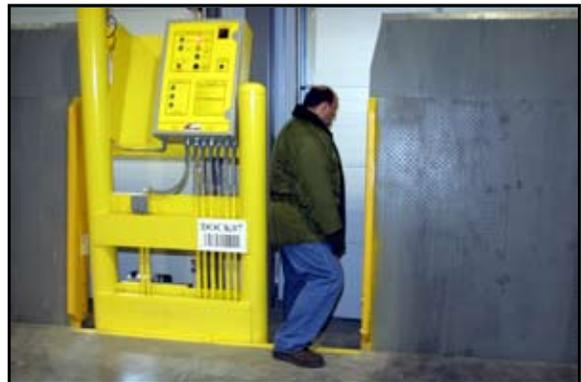
Proper bollard/control stanchion design and placement controls access to the pit area. Where power doors are utilized, restricted access to the pit area can be accomplished by widening control stanchions.
