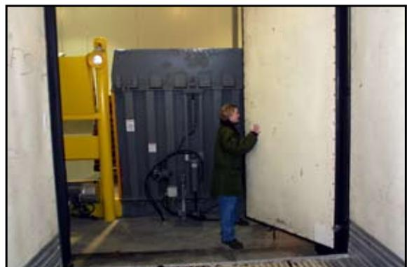
A continuous pit is ideal when opening trailer doors into the building, a desirable application consideration for enhanced environmental and security control.
