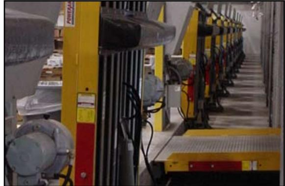
Individual pits can be formed by notching around door jambs to allow the door to close firmly to pit floor, creating room for staging between pits. A continuous pit is more economical to construct and permits easy access for house keeping.
