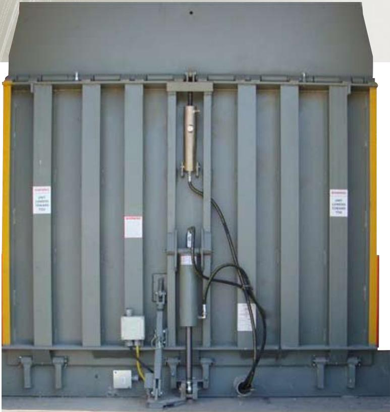
VS shown with remote motor and solenoids
