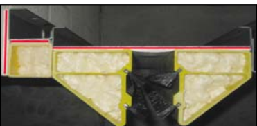
Thermal breaks (red highlights) in side column.
