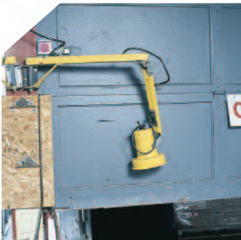
Old technology truck lights are prone to damage from overhead doors and fork lifts.
